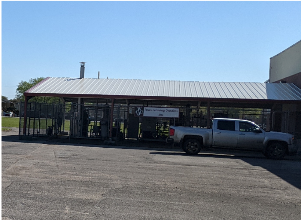
Figure 3 – Steel-Framed Open Canopy Structure at North Side of Building
